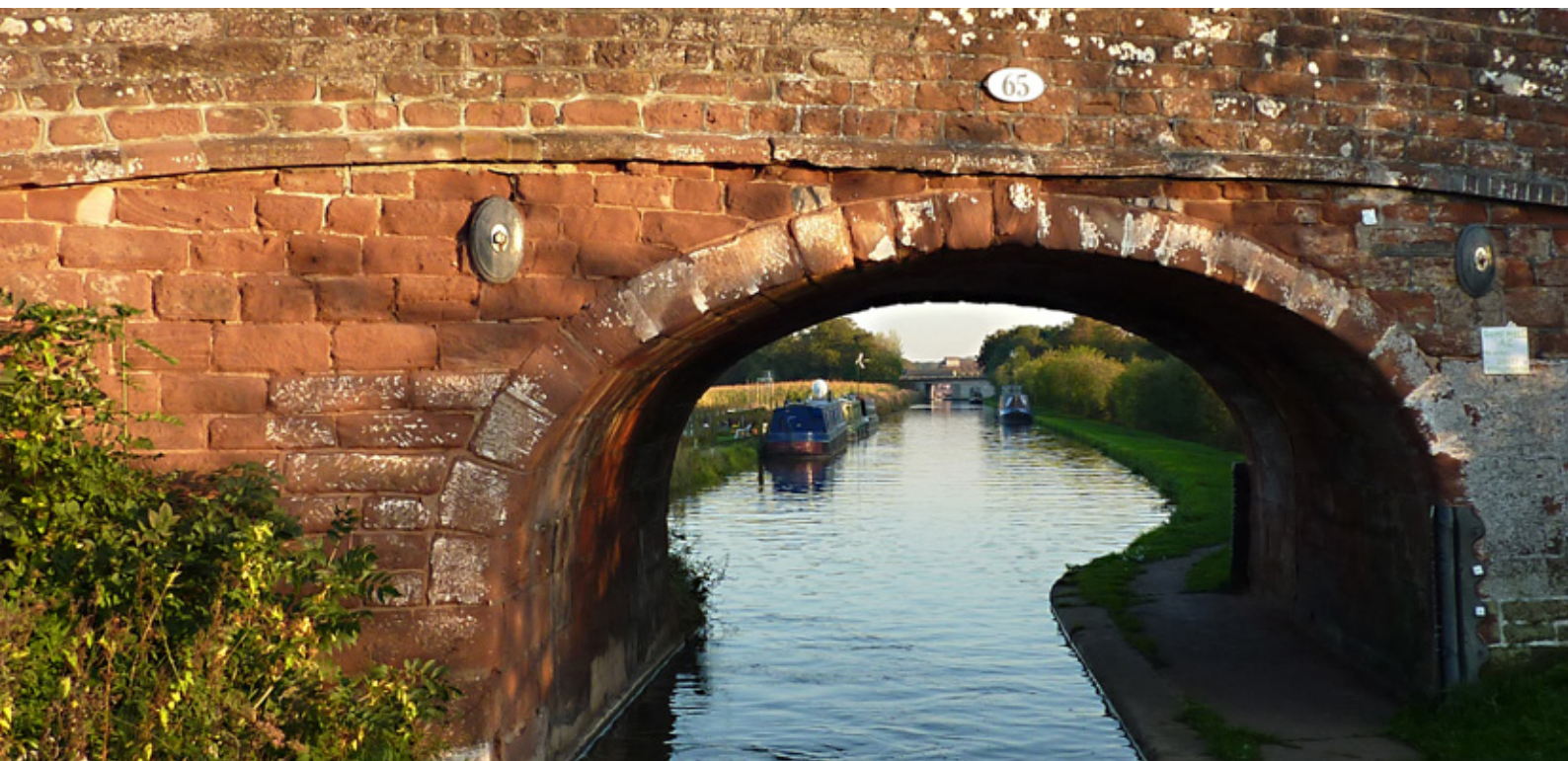
Local sandstones were used for bridges on the Shropshire Union Canal. ©Julie Harrald.
